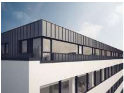
Close-up Image of the 'Zinc' clad Penthouses
